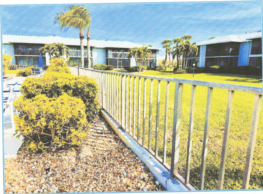
NORTH POOL ENCLOSURE
