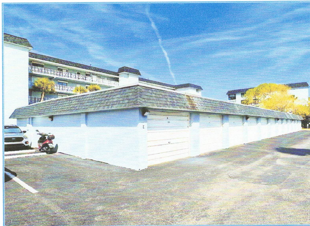
GARAGE E, SOUTHEAST CORNER
