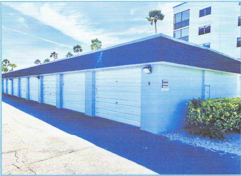
GARAGE B, NORTHWEST CORNER
