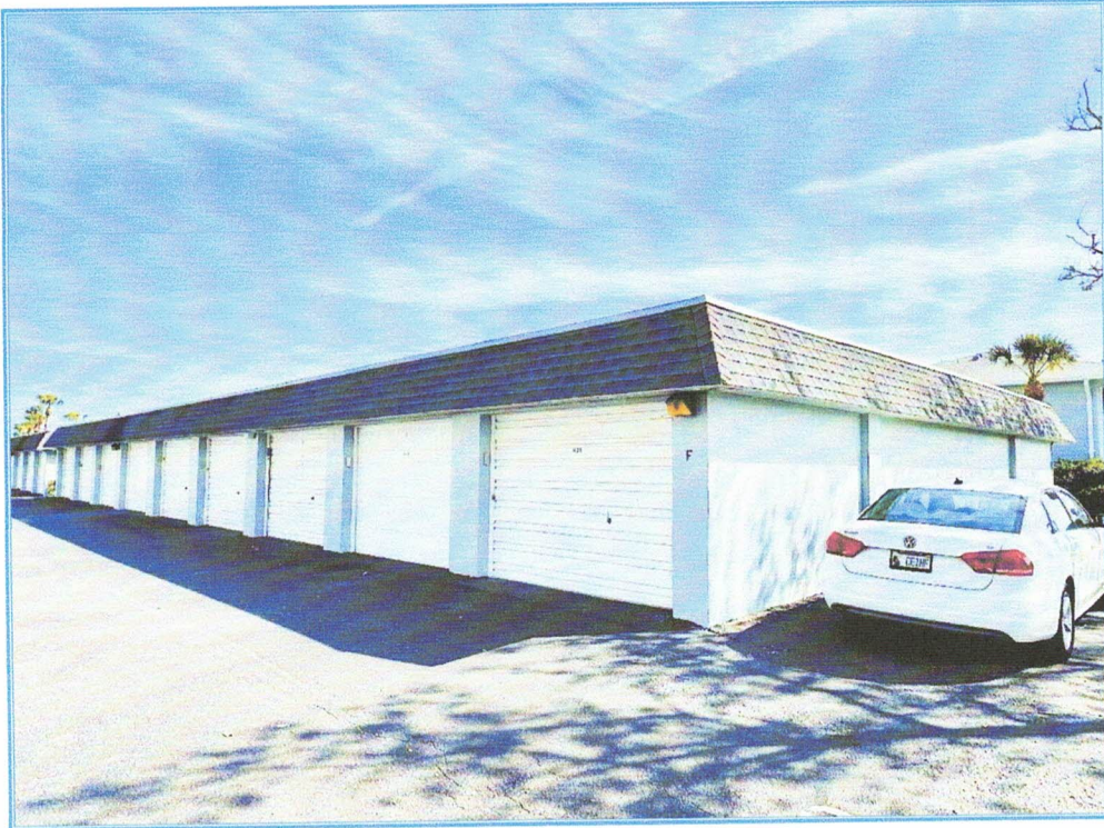
GARAGE F, SOUTHWEST CORNER
