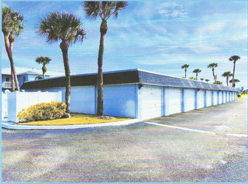
GARAGE A, SOUTHWEST CORNER
