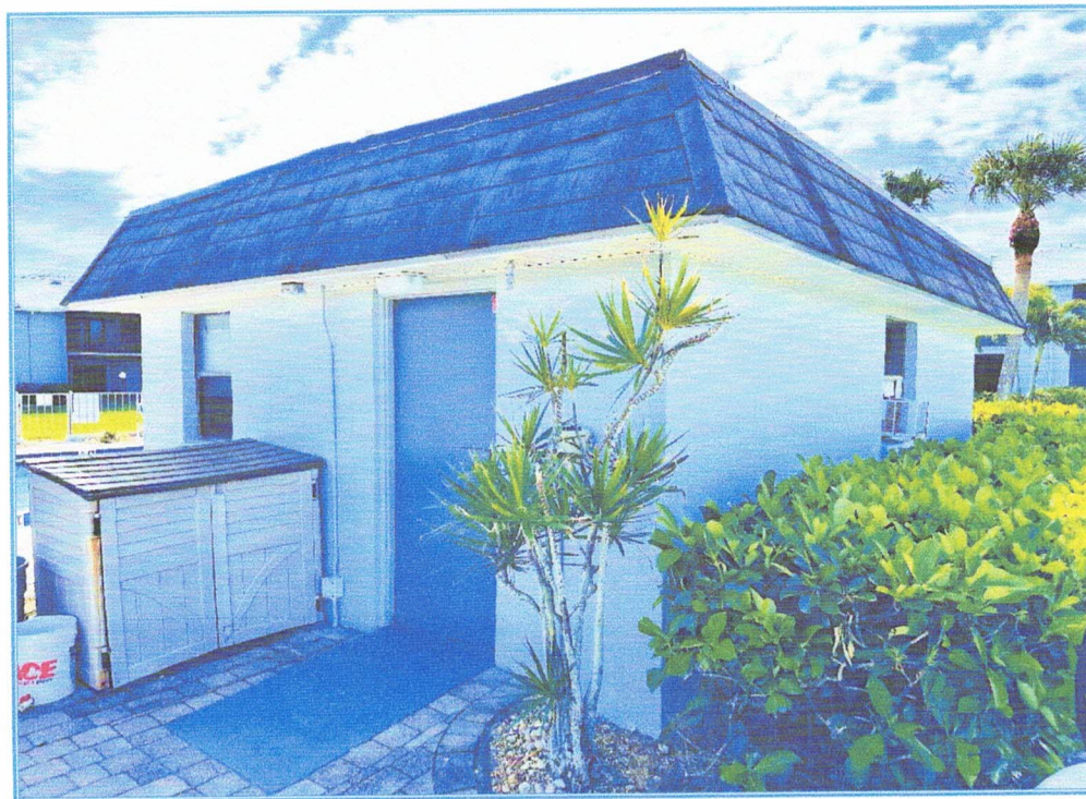
NORTH POOL BATHHOUSE, NORTHWEST CORNER
