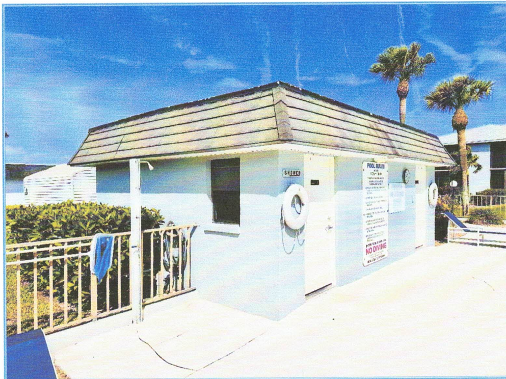
NORTH POOL BATHHOUSE, SOUTHEAST CORNER
