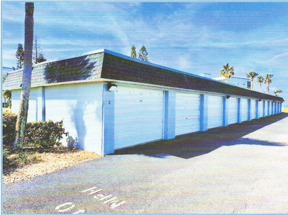
GARAGE C, NORTHEAST CORNER
