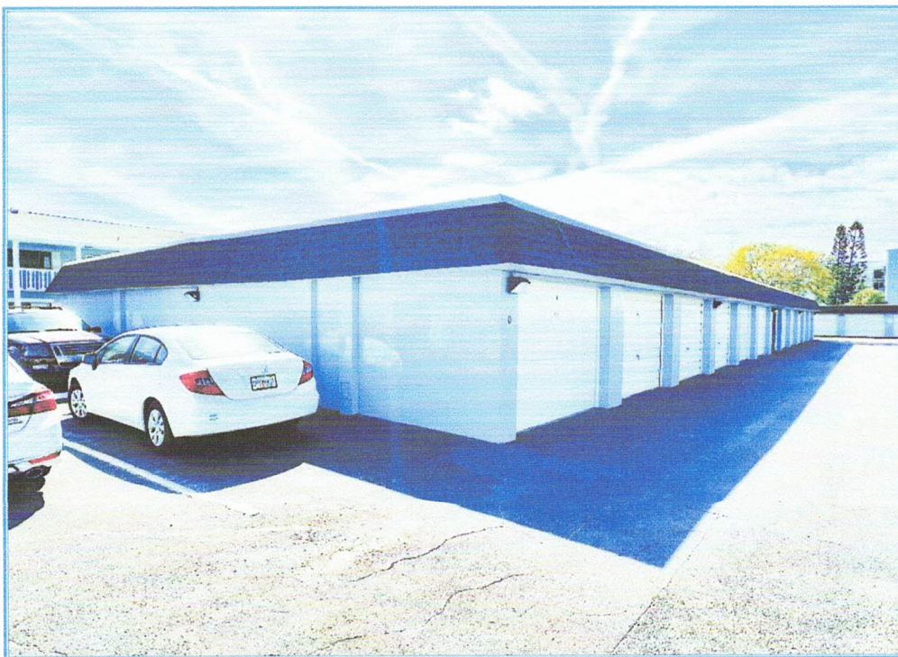
GARAGE D, NORTHWEST CORNER
