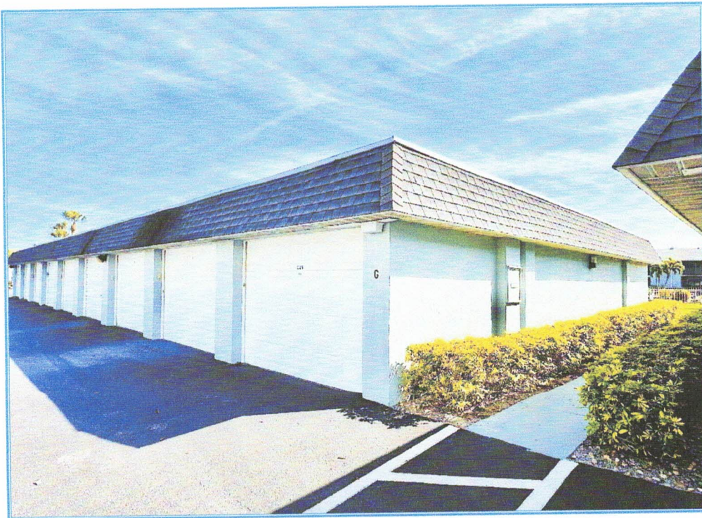
GARAGE G, SOUTHWEST CORNER
