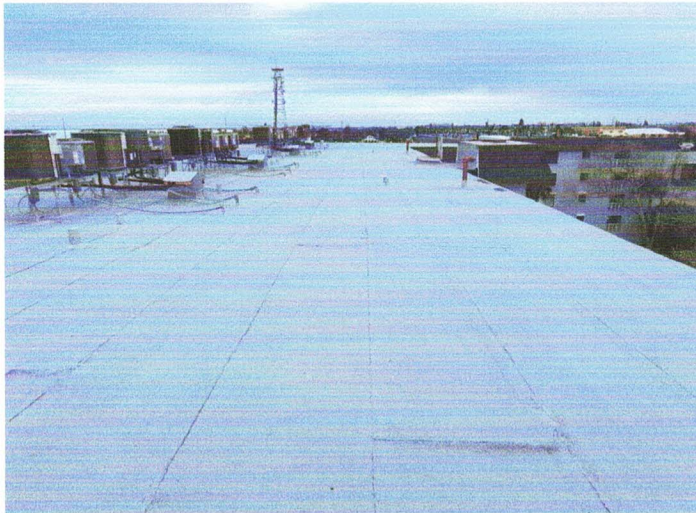
Overview of a completed GAF modified roof system on building 9.
