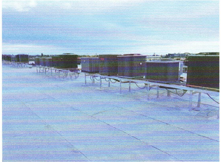
Overview of a completed GAF Modified roof system on building 8.
