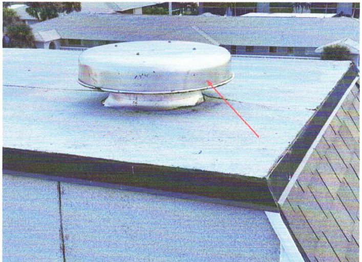
New vents installed to replace existing elevator and trash roof vents.
