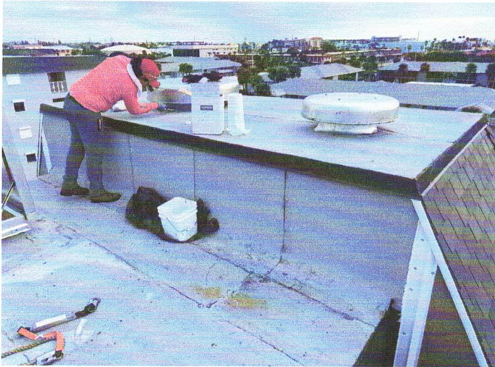
In progress liquid reinforced flashing of new rooftop vents.
