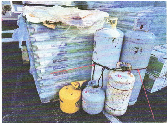
Large propane cylinders are secured in storage on the ground.
