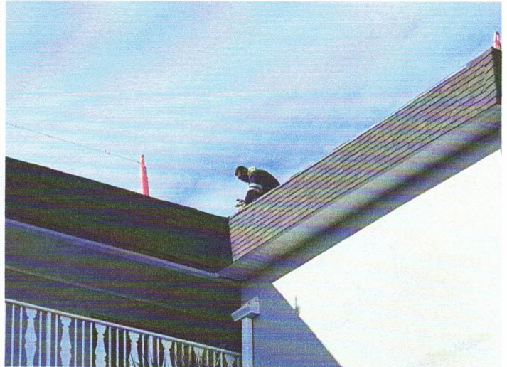
Metal cleat installation continues on the low slope perimeter roof.
