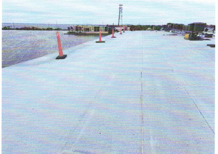
Completed roof section of the GAF granulated modified roofing.
