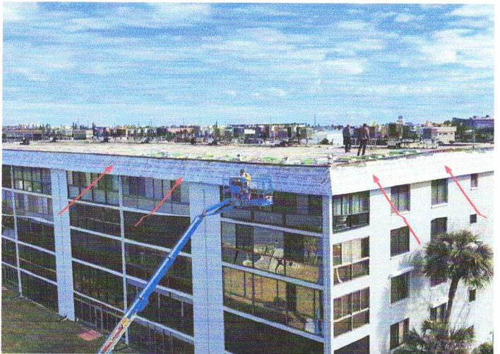
In progress installation of the self-adhering underlayment continues.
