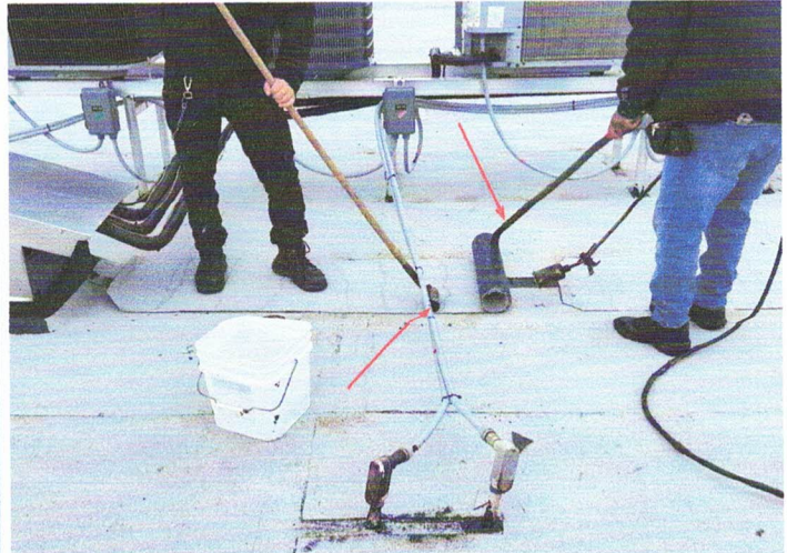
Red arrows indicate stick roller and pull stick being used during the torch operations.
