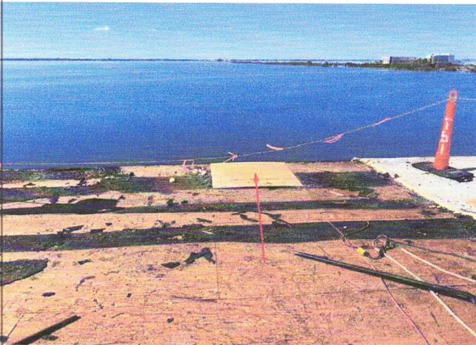
In progress new plywood sheathing installation.
