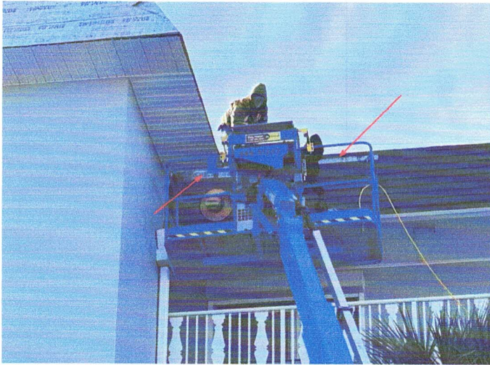
Shingles being installed from the manlift.
