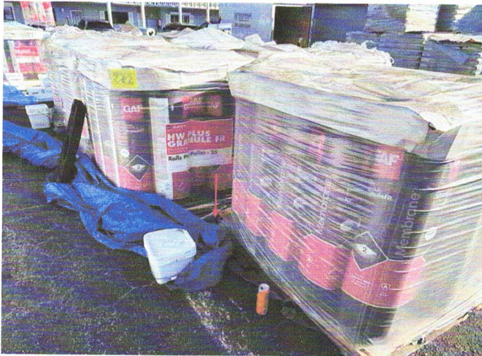
Project specific GAF materials stored in their original wrappers.
