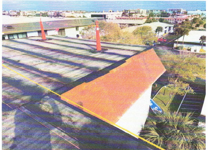
Rooftop view of the plywood sheathing at the mansard.
