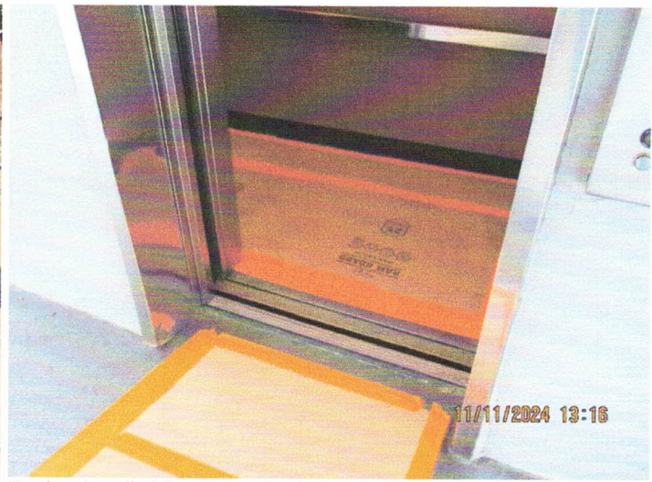
Roofers installed floor protection in the elevator and between the elevator and roof access ladder.
