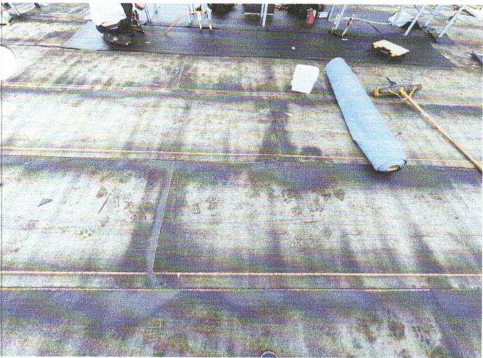
View showing proper staggering of the modified roll end laps.
