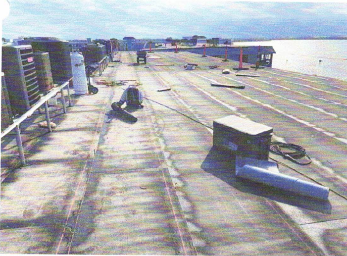
All modified bitumen roofing has been installed per manufacturer specifications and per the Keystone Engineering project manual.
