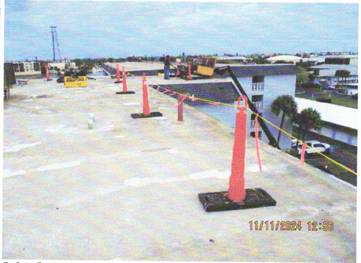
Safety flags staged around the roof perimeters.
