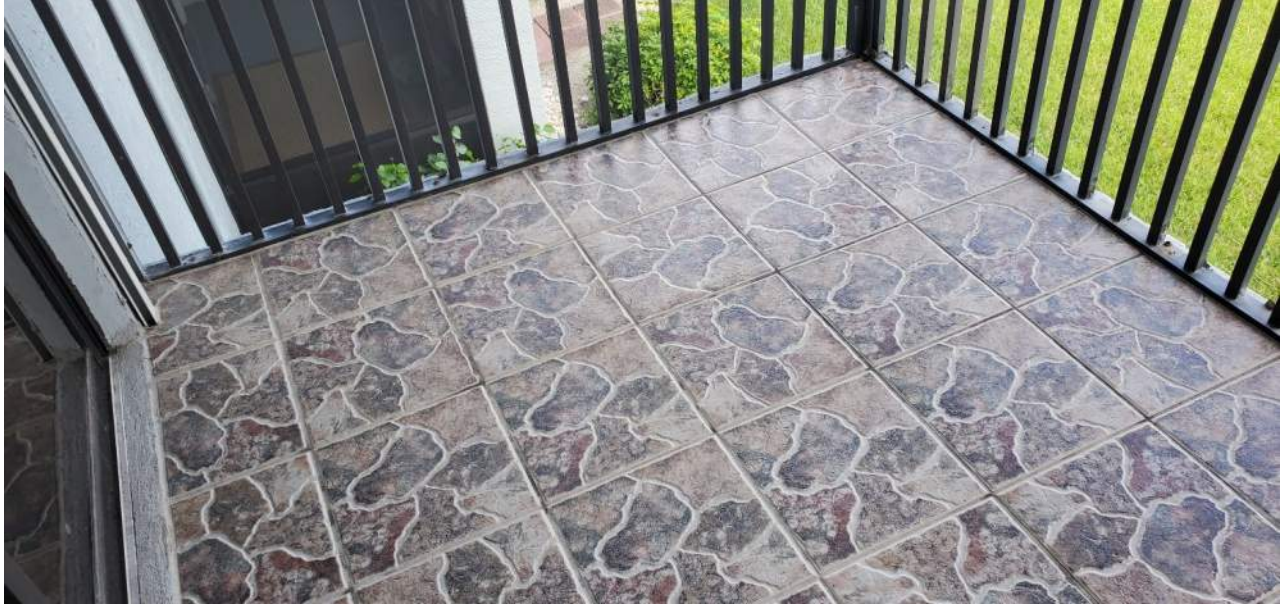
Example view of concrete slab with tiles
