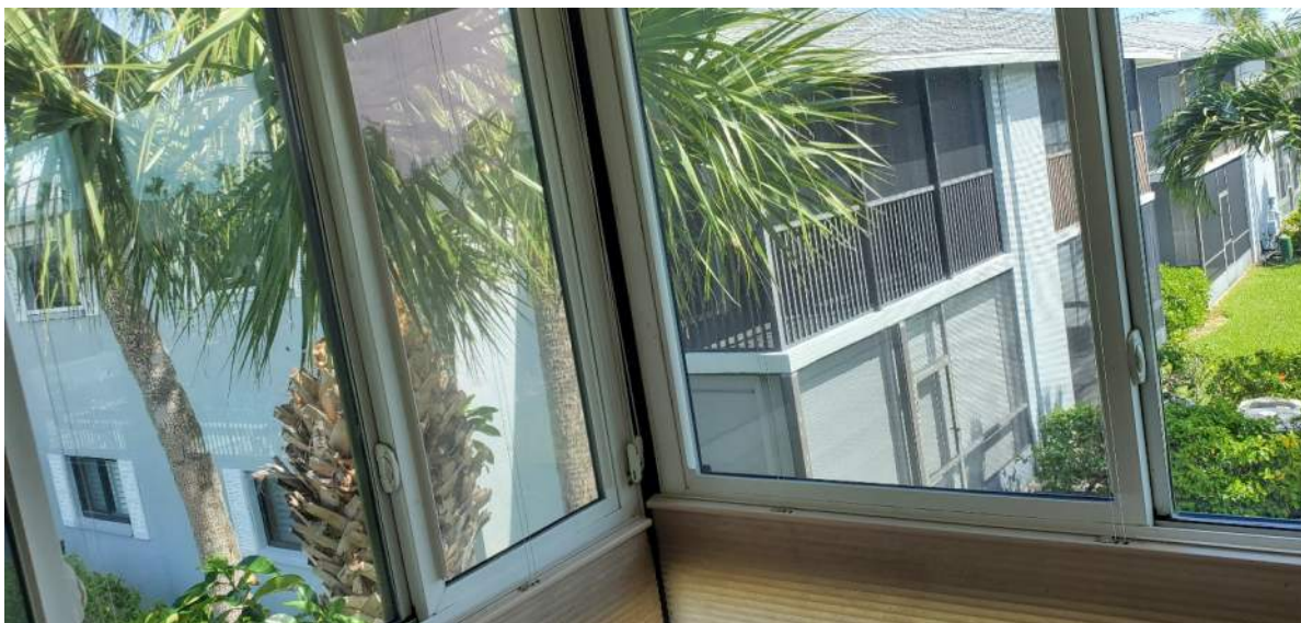
Example view of porch with glass enclosure
