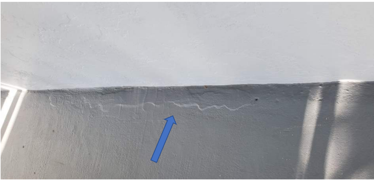
Example view of spalling concrete on walkway
