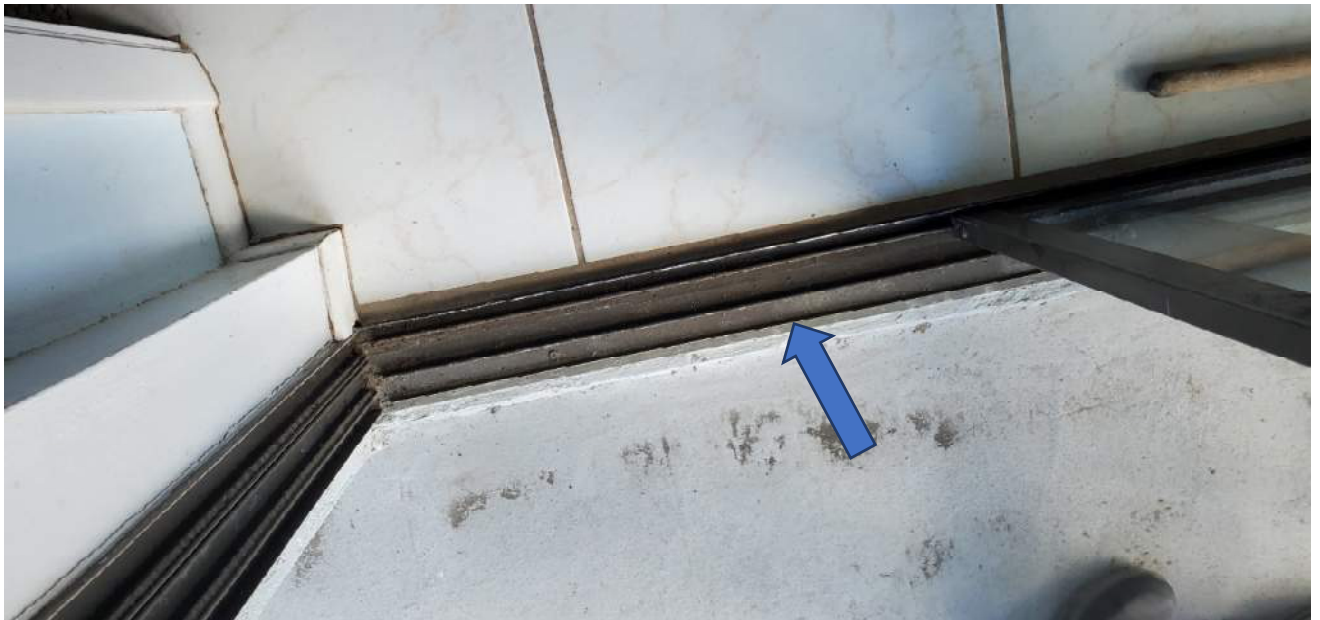
Example view of rusting sliders.
