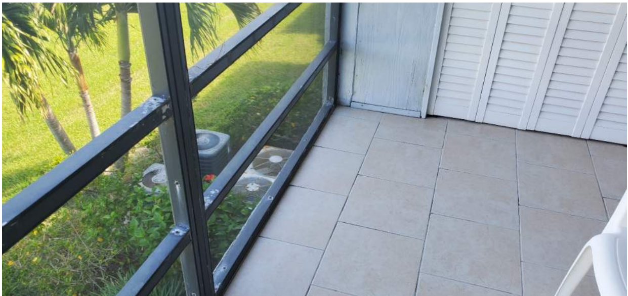
Example view of peeling screen railings and tiled slab. Note the old style type screens without pickets
